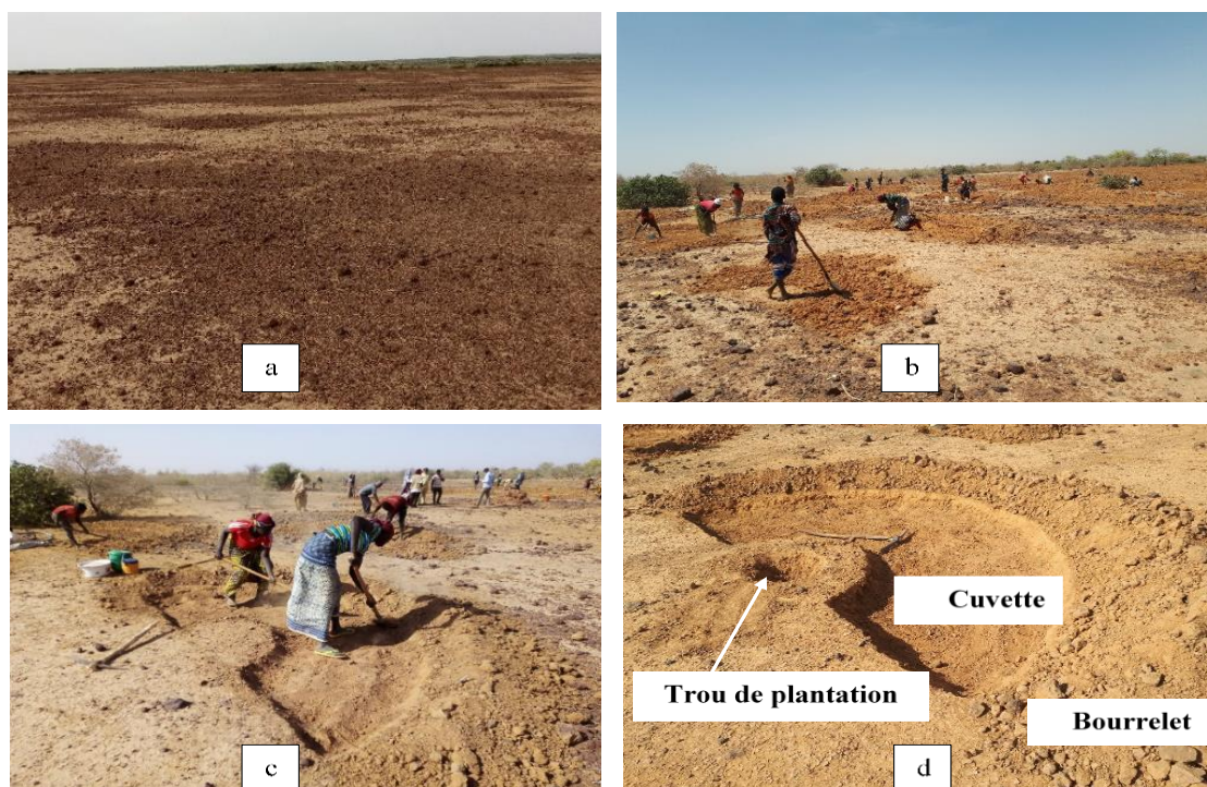
Fig. 2: Construction of the half-pipe: a: Undeveloped area; b: the first diggings following the tracing; c: construction at an advanced level and d: Ready-made half-moon
